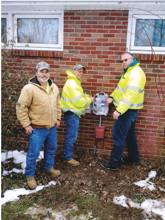
Town of Pendleton Water/Sewer Superintendent Jim Argo (far left), along with Pendleton Field Technicians Jeff Jarvis (center) and Rick Geltz (right), with one of the Town's 400 E/One Upgrade grinder pump control panels.
