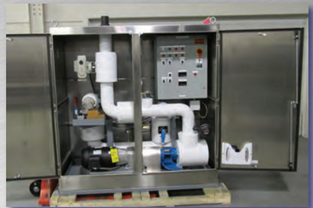
Weather proof, free standing SS cabinet (interior).
