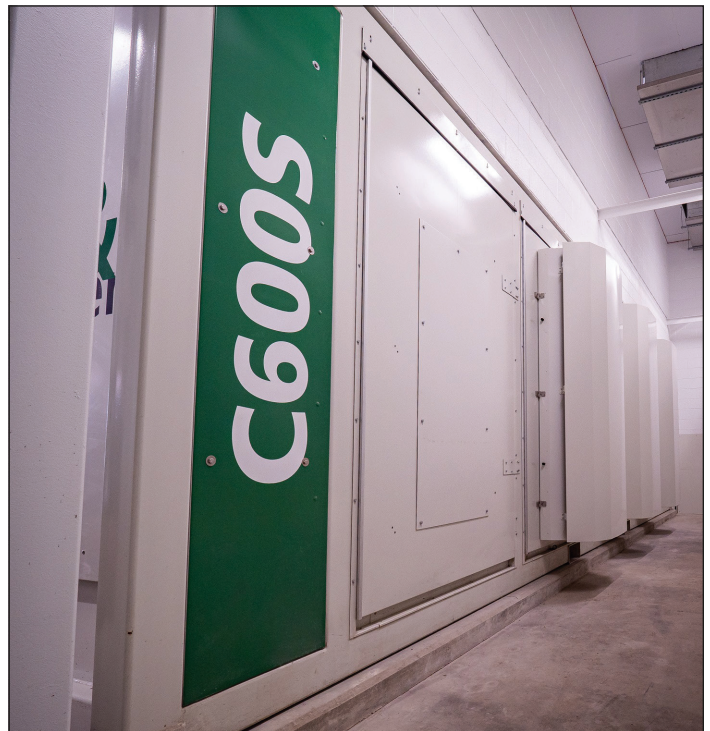
Capstone 600kW microturbine supplied by GEM Energy at the Oneida County WPCP.
