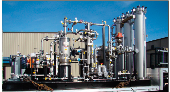
Digester gas conditioning skid by Unison Solutions at the Oneida County WPCP.
