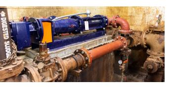
Seepex Smart Conveying Technology means quick and easy disassembly. The top half of the stator can be removed to gain access for visual inspection of rotor and stator and easy blockage removal. Fulton WWTP also has the Seepex Dry Running Protection Device TSE, which monitors the temperature of the stator and alarms when the set limit is reached.
