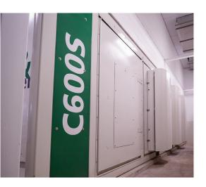
The CHP system is generating 50-60% of the plant's electrical power. The plan is to produce more power once the project is completed and the CHP is expanded.
